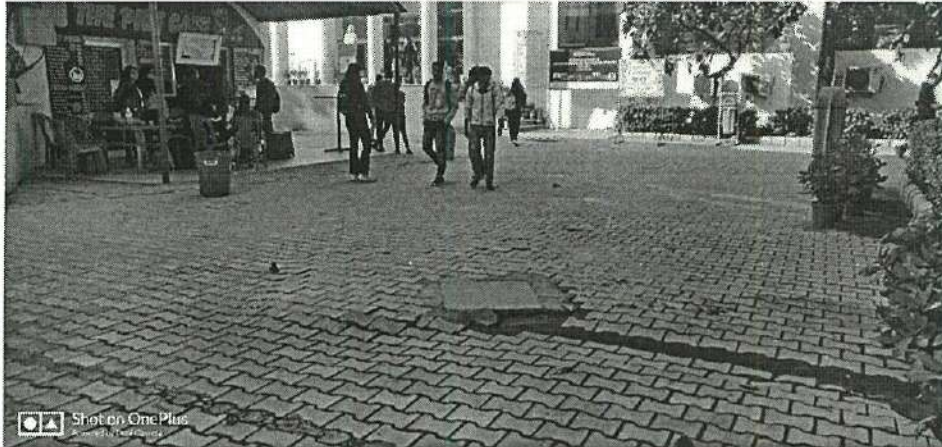
Underground tank for rainwater harvesting adjacent to institute Canteen, D and E Blocks
